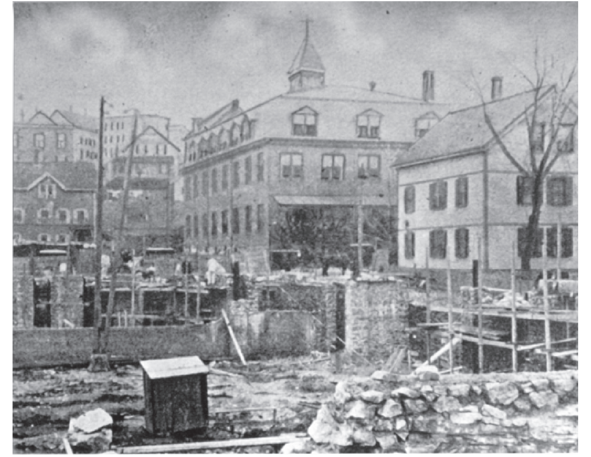
1914 Saint Ann's church on Cumberland Street. Construction photo. Ground broken November 11, 1913.
